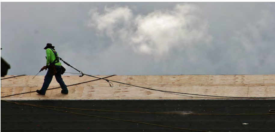
Top photo: Workers covered the back room of the auditorium with a blue tarp for protection. Bottom photo: A tethered for safety roofer prepares plywood for its tarpaper layer.
